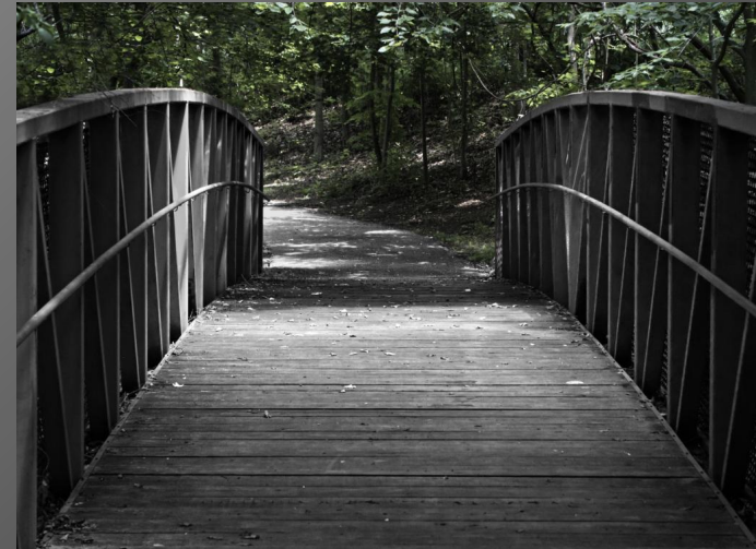
Louis Sapienza Bridge in Woods
